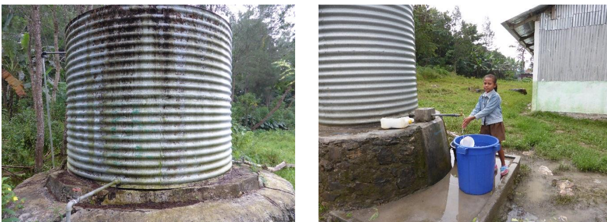
Figure 13 – EBC Mundo Perdido tanks – rusted upper toilet block tank (left) and kitchen tank (right)
