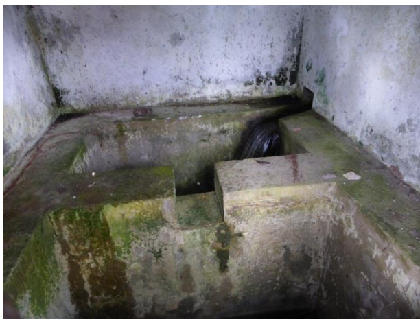
Figure 5 – Uaibua Spring intake
