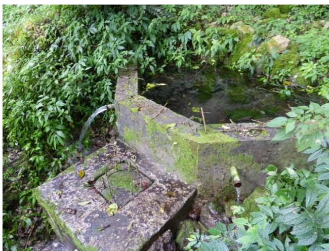
Figure 4 – Uaiquirona Spring intake
